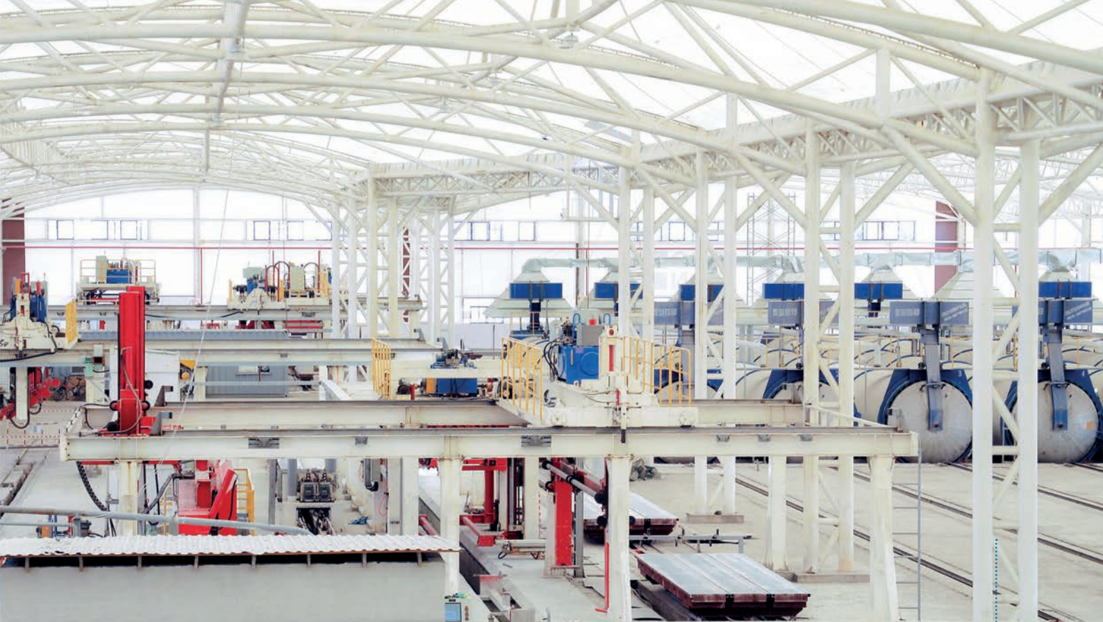
Interior overview of the new plant.
